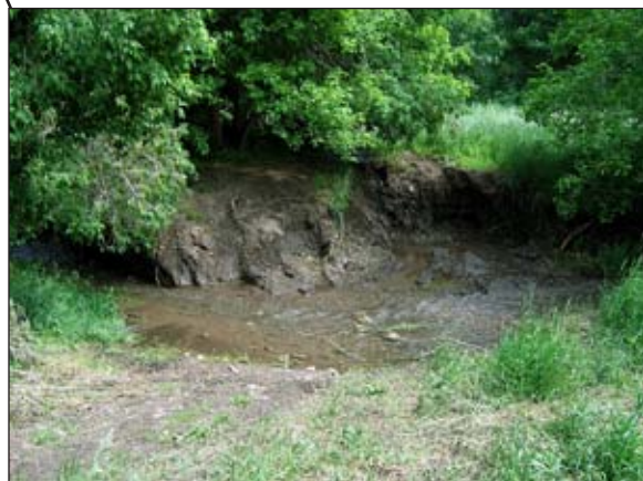
“Digging” across a streambed
