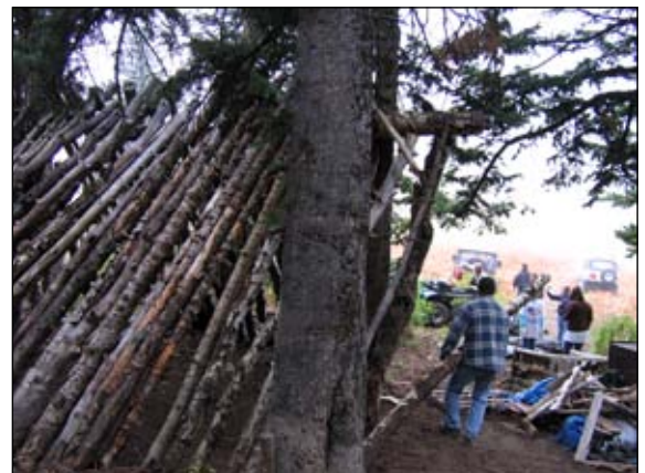
remove a lean-to and garbage, 2004.
