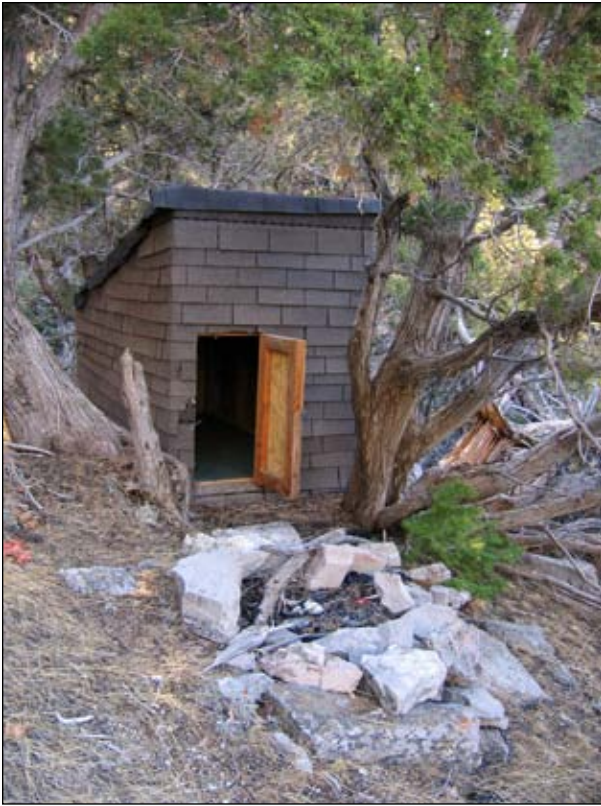
Logan Dry Canyon illegal structure before...
