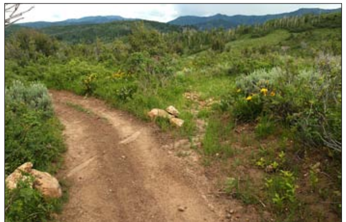
Water diversions were installed and are working.
