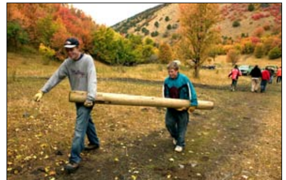
Volunteers build fence in Millville Canyon and...
