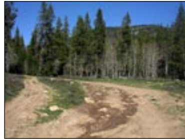
R-3 Wider than typical
